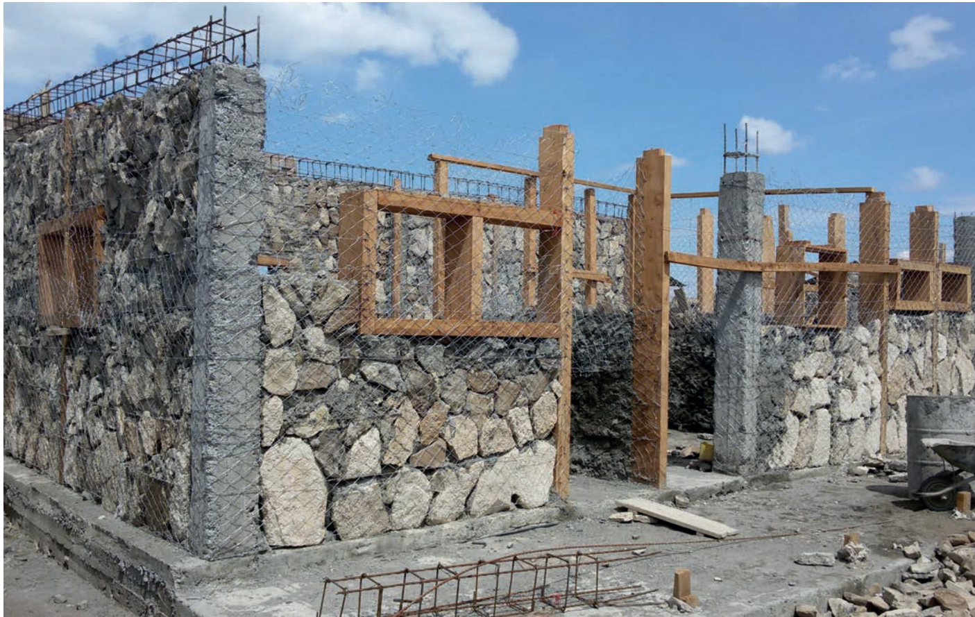
↑ Fig. 15 The M&C Centre under construction using local limestone for the walls. (Photo: L. Beninati).
