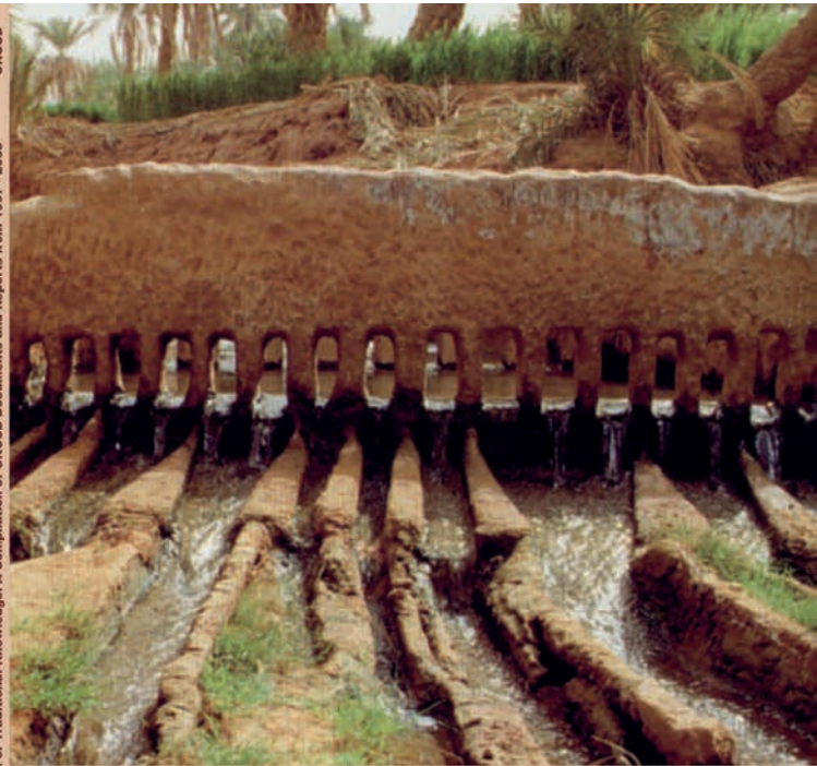
Oasis of Timimeun (Algerian Sahara), kesria, a water quota sharing system. Photo: P. Laureano.
